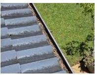
Some sections of guttering show signs of rust and require repair / painting with Killrust or better.
